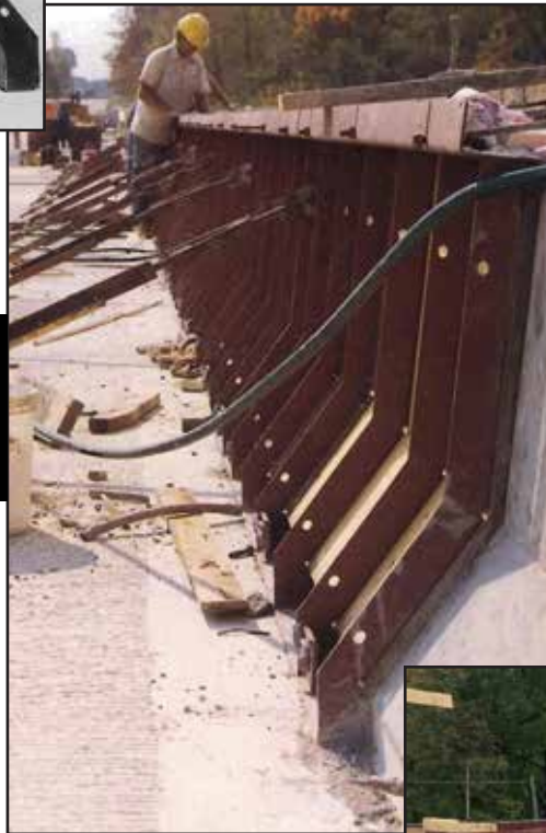
BARRIER/PARAPET WALL FORM
